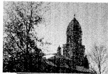
Lewiston City Building constructed in 1892
